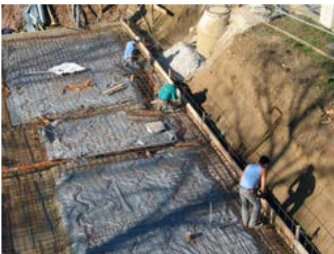
Construction zone, new foundations forming
